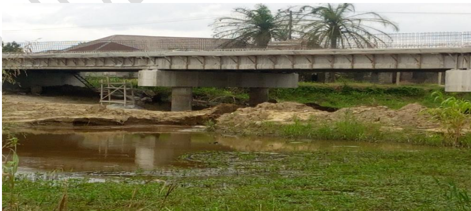
Plate 2. Ongoing Bridge Constructions in the Kolo Creek
