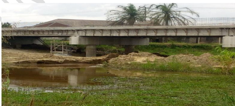
Plate 2. Ongoing Bridge Constructions in the Kolo Creek
