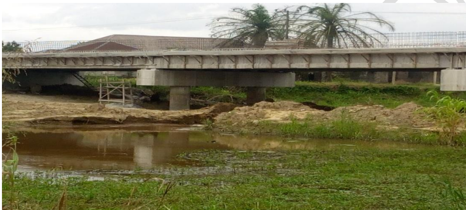
Figure 3. Ongoing Bridge Constructions in the Kolo Creek
