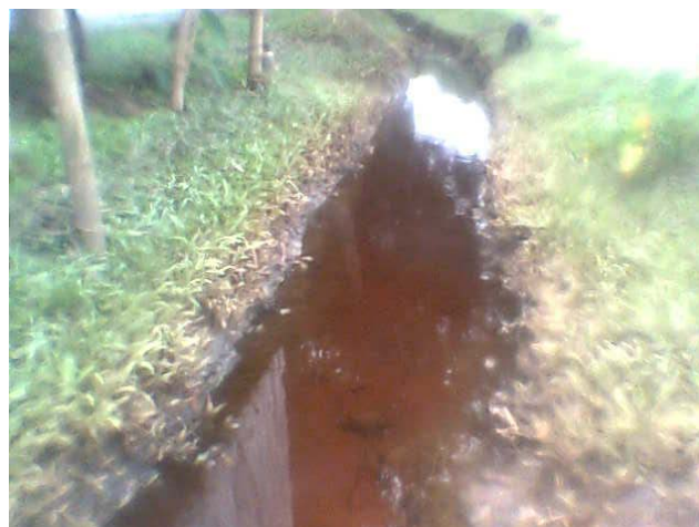
99 Figure 3: Drain water from coal stockpile area
