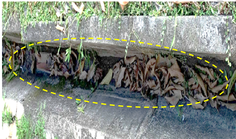
Figure 8: Accumulation of leaves inside the drain
