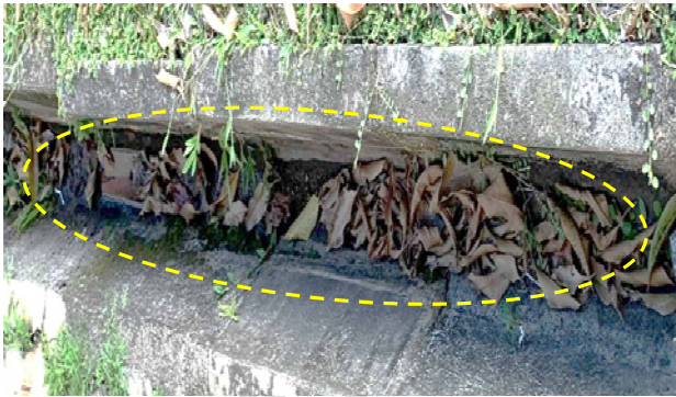
Figure 8: Accumulation of leaves inside the drain
