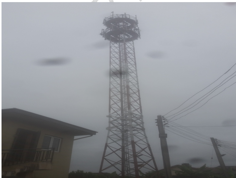
Figure 2. Picture of Airtel Mast Visited at Akwaka
