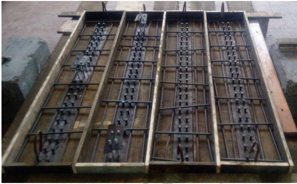
b- Wooden form and reinforcement of concrete slab
