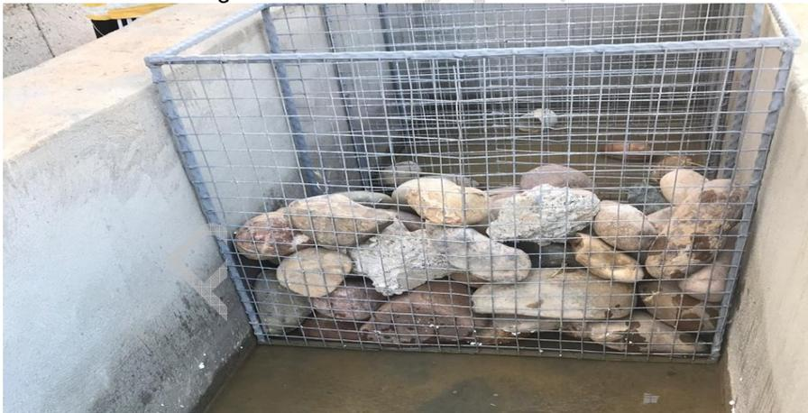
**Fig.13. Interceptor dike to control the erosion**
