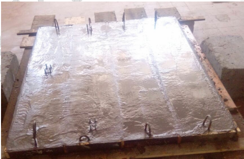
c-Casting of R.C. slab
