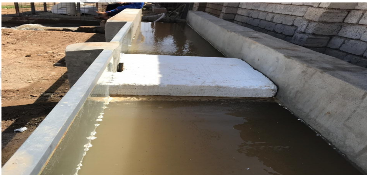
Fig. 4. The Floating Brige construction
