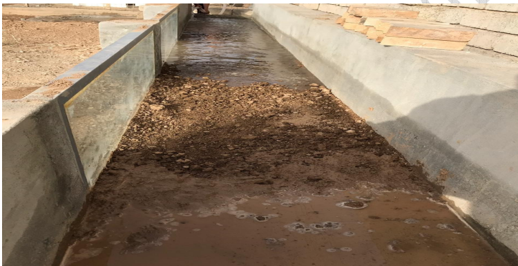
Fig. 1. Erosion control through stabilizing the area of the waterway
