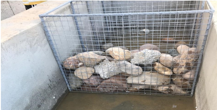
Fig.13. Interceptor dike to dike to control the erosion
