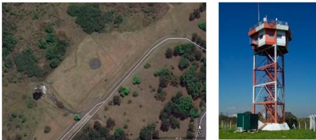
Fig. 2 – Aerial and ground view of the tower ACA and his environmental field region
