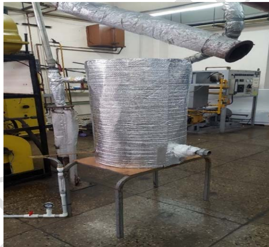
Figure 14: Experimental set up - Waste Heat Recovery from Diesel Engine
