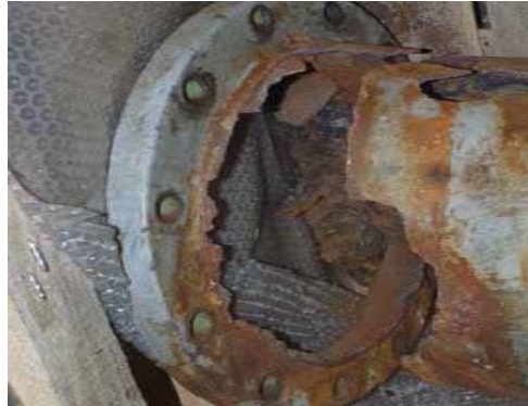
Fig. 1. Corroded Piping System
