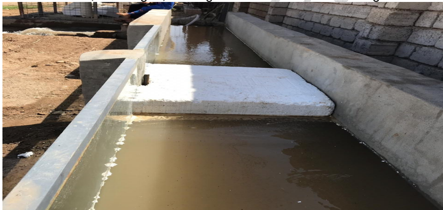
Fig. 4. The Floating Bridge construction
