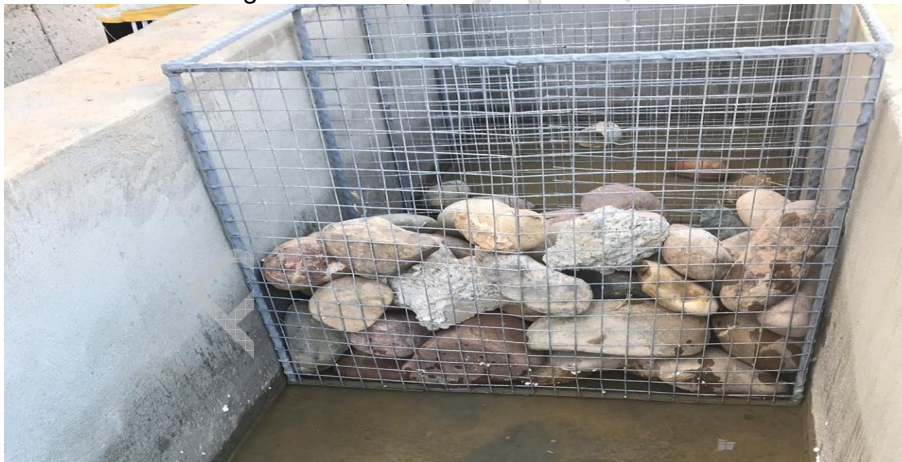
Fig.13. Interceptor dike to control the erosion
