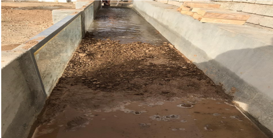
Fig. 1. Erosion control through stabilizing the area of the waterway
