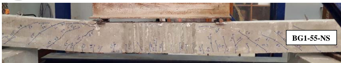
Fig. 6d. Typical ductile flexural failure for strengthened beams
