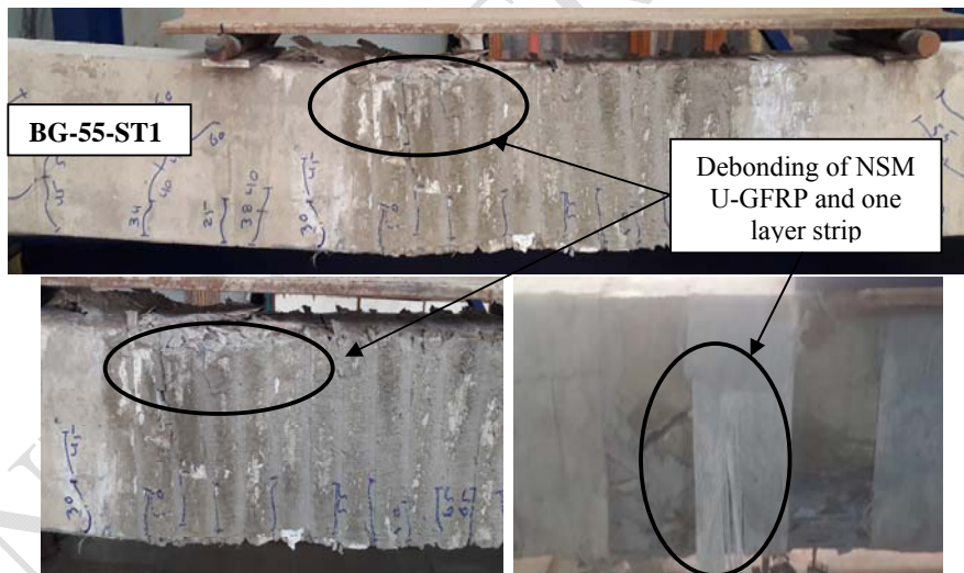
Fig. 6c. Typical de-bonding/flexural failure
