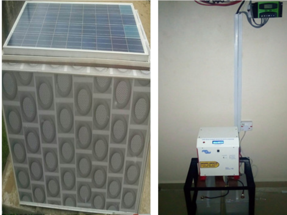
a). Solar panel on a platform 1m high.b). Grid connection
