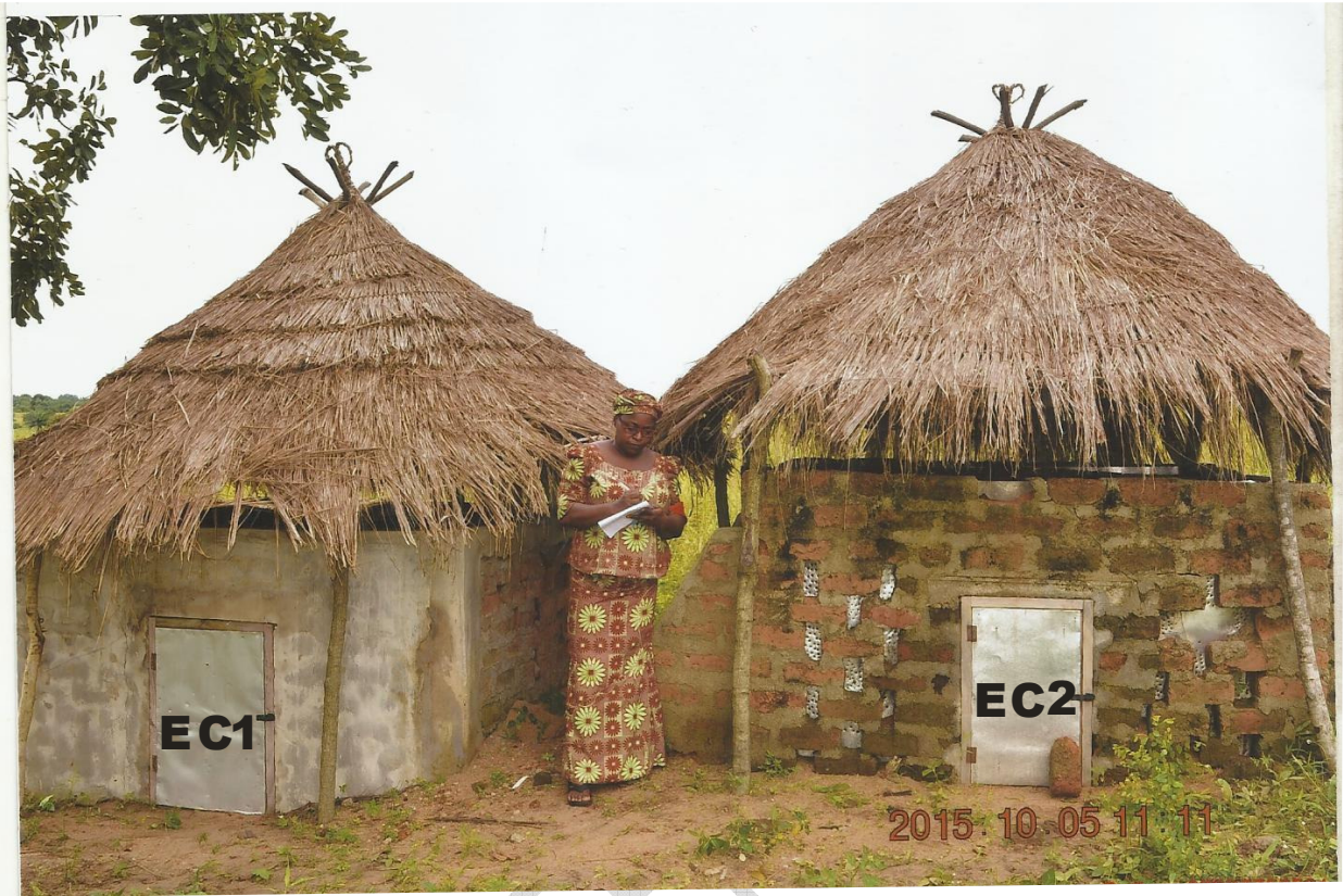
Plate 1: Evaporative Coolers 1 & 2
