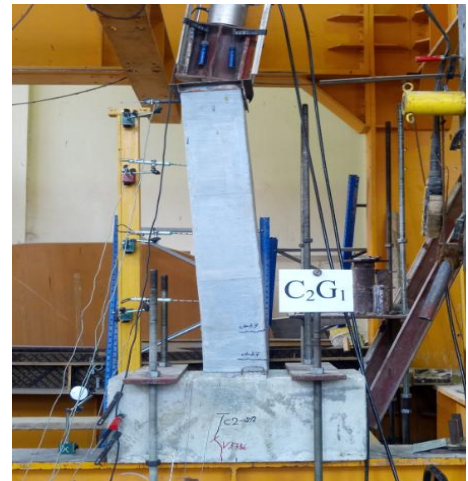
Figure 10: The cracks of column C2G1 at failure under the ultimate axial load
