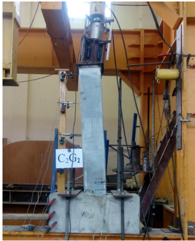
Figure 8: The cracks of column C2G2 at failure under the ultimate axial load
