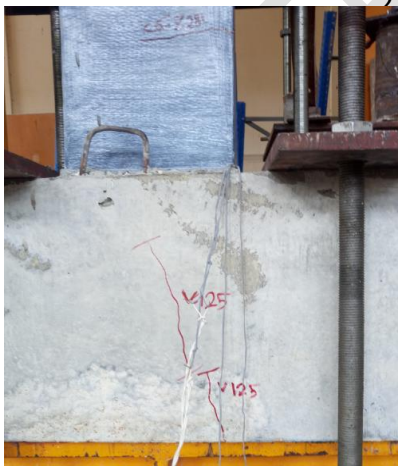
Figure 12: The cracks of column C2C1 at failure under the ultimate axial load
