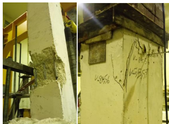
Figure 7: The cracks of column C2 at failure under the ultimate axial load
