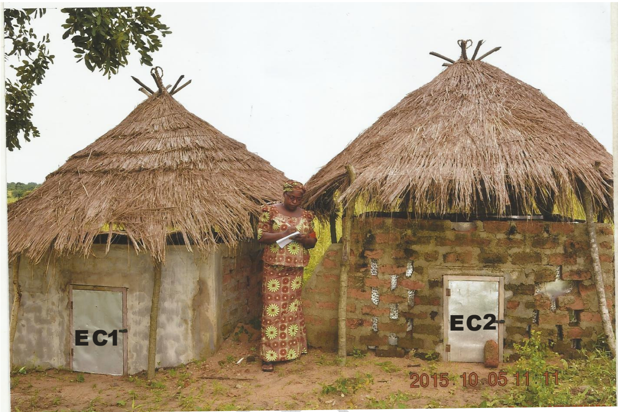
Plate 1: Evaporative Coolers 1 & 2
