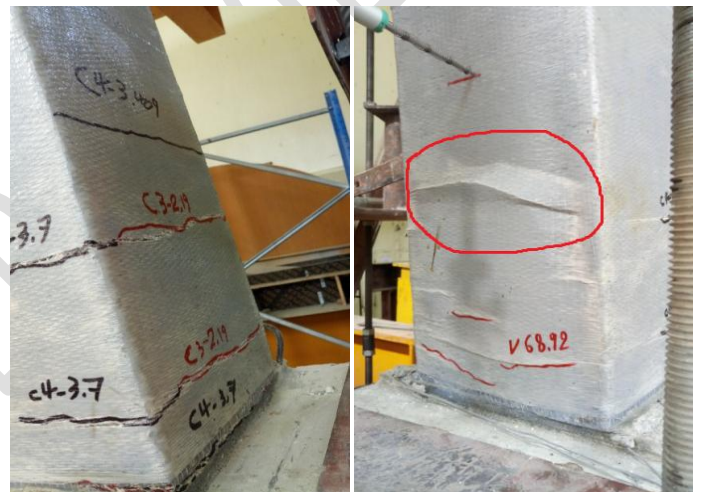
Figure 10: The cracks of C2G1 column at failure under the lateral load. Separation of the fiber is noticed.
