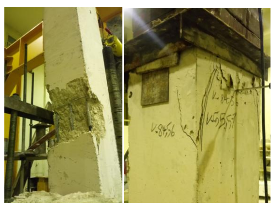
200 201 Figure 7: The cracks of column C2 at failure under the ultimate axial load
