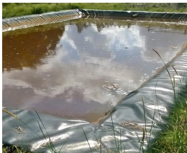
Fig.1. Settling pond of SIW leachates
