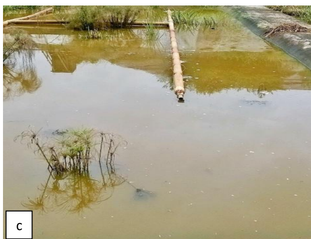
Fig. 8. Progressive disappearance of plants in planted filters: a) PF1 at 1 day b) PF1 at 2 months c) PF1 at 3 months
