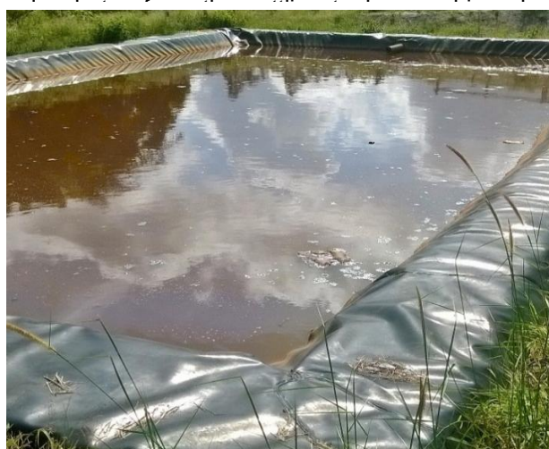
Fig.1. Settling pond of SIW leachates
